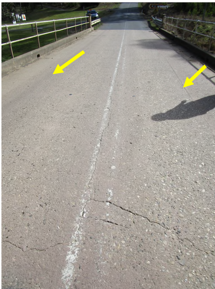
Photo 17. Transverse cracks in centre portion of deck. Note longitudinal construction joints (arrowed)
