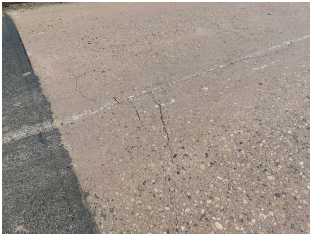
Photo 18. Transverse cracks in deck near east abutment.
