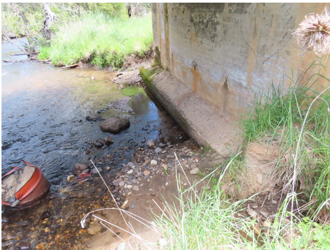
Photo 20. West abutment with slight erosion.
