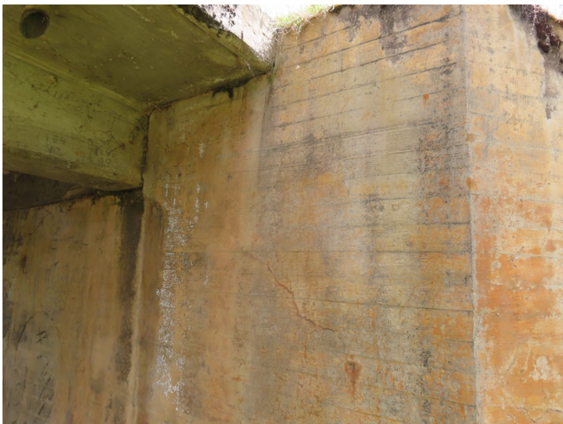
Photo 12. Typical crack in wingwall/abutment
