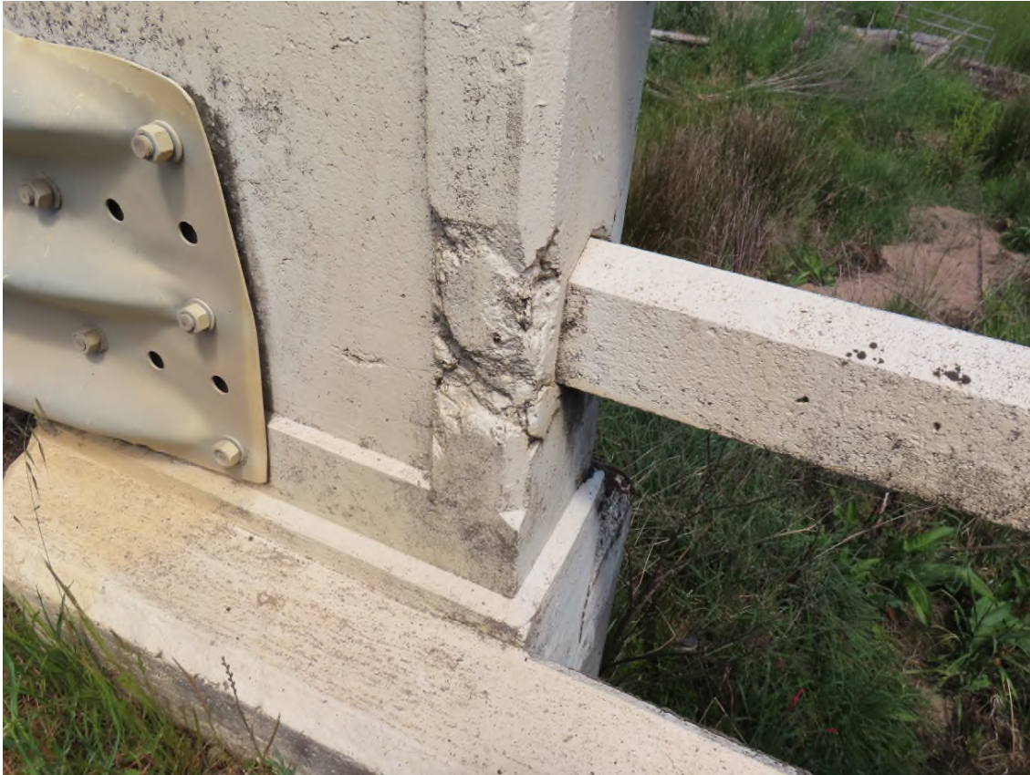
Photo 5. Minor damage to bridge rail post.
