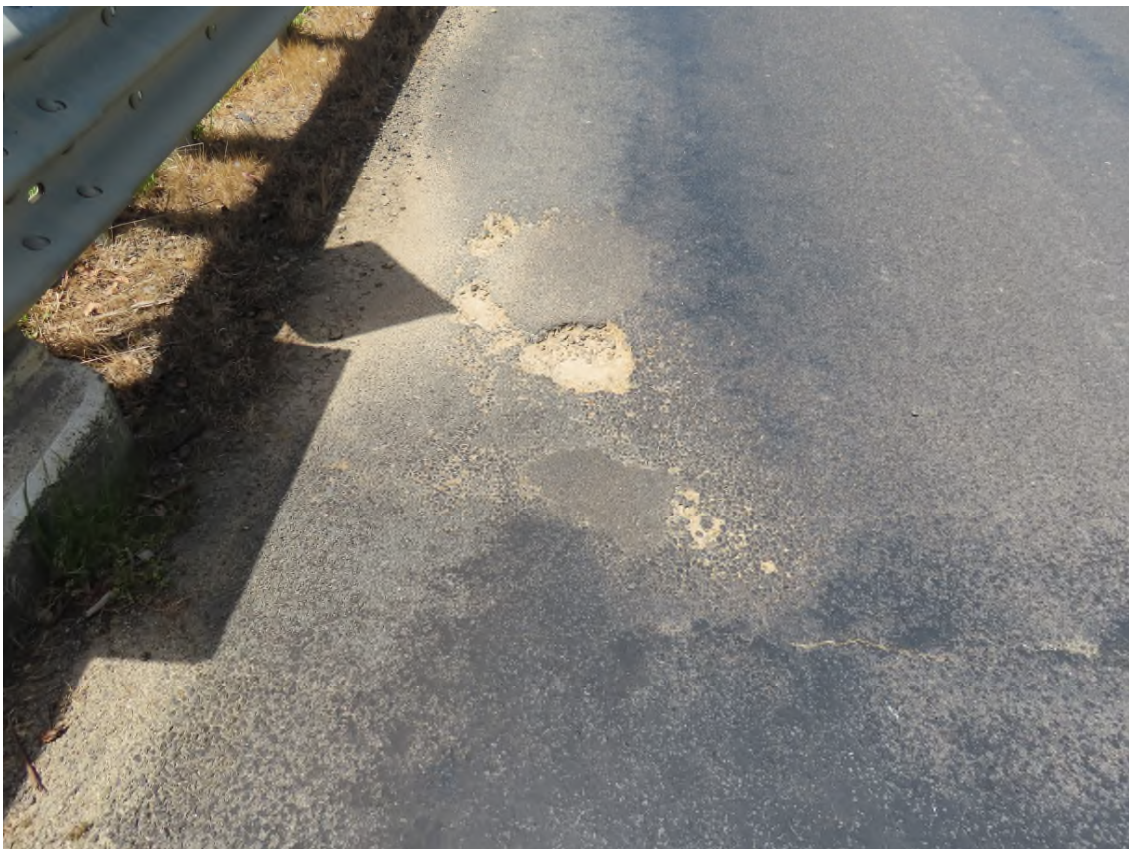
Photo 6. Pot hole at end of deck in road surfacing east end, north side.
