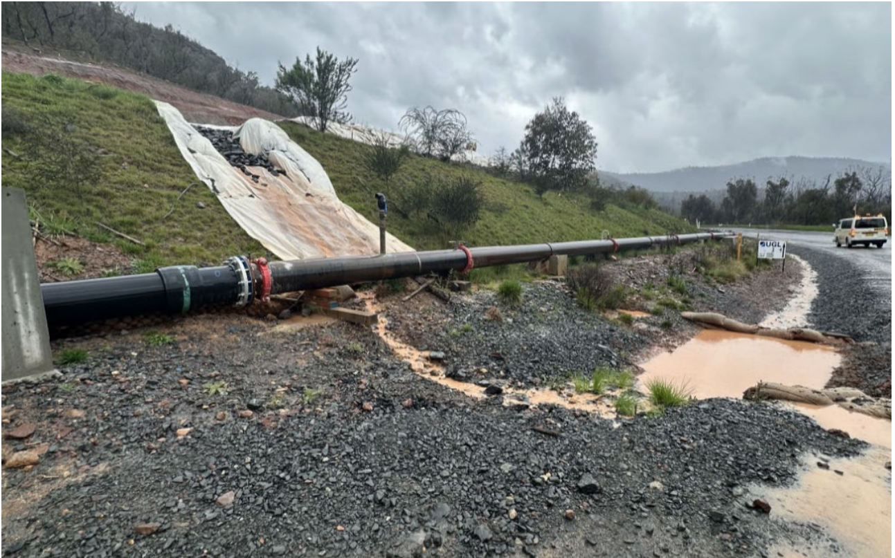
Plate 7: Erosion and sediment control devices e.g. rock checks and sandbagging installed within Track 8 (25/09/2024).
