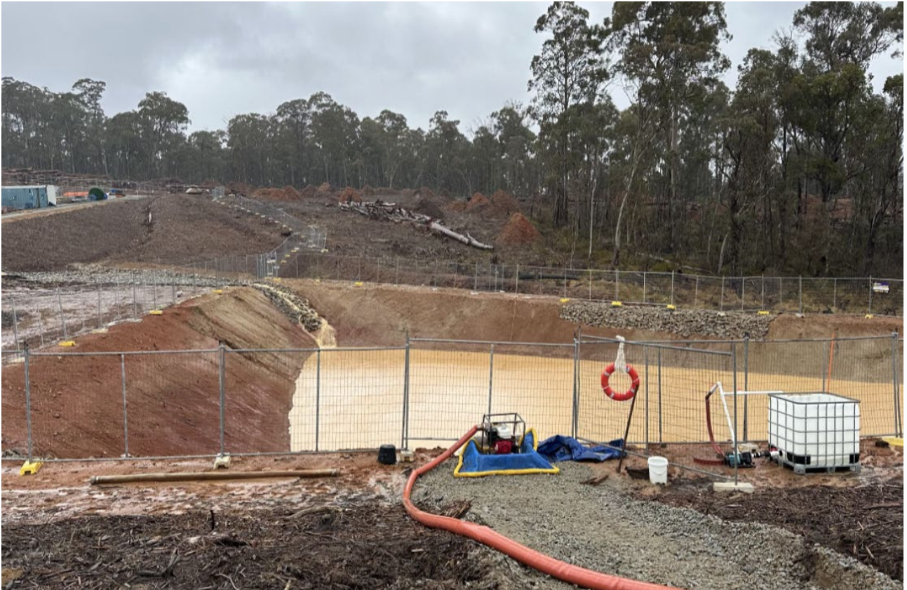
Plate 13: Sediment basin located within Maragle Substation Project Area (25/09/2024).
