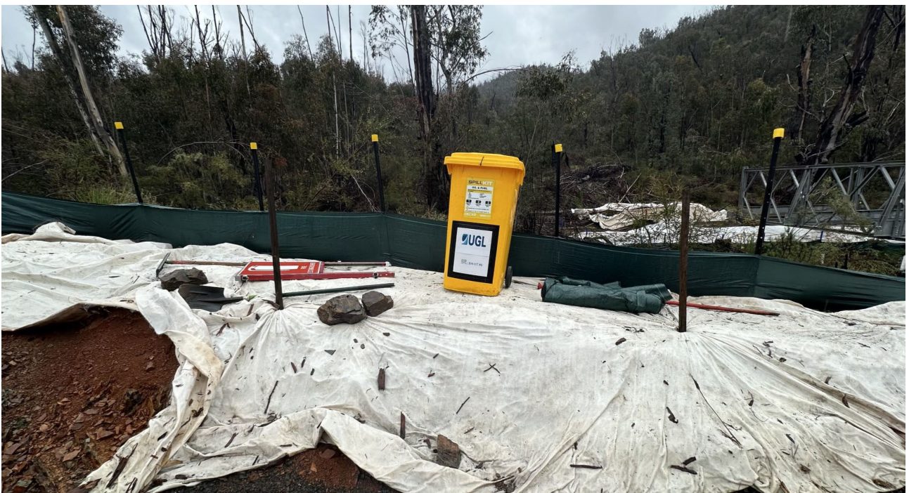
Plate 7: Erosion and sediment control devices e.g. rock checks and sandbagging installed within Track 8 (25/09/2024).
