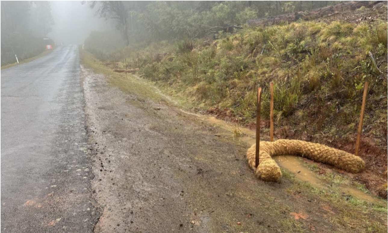
Plate 5: Erosion and sediment control devices e.g. coir logs installed alongside roadside (25/09/2024).
