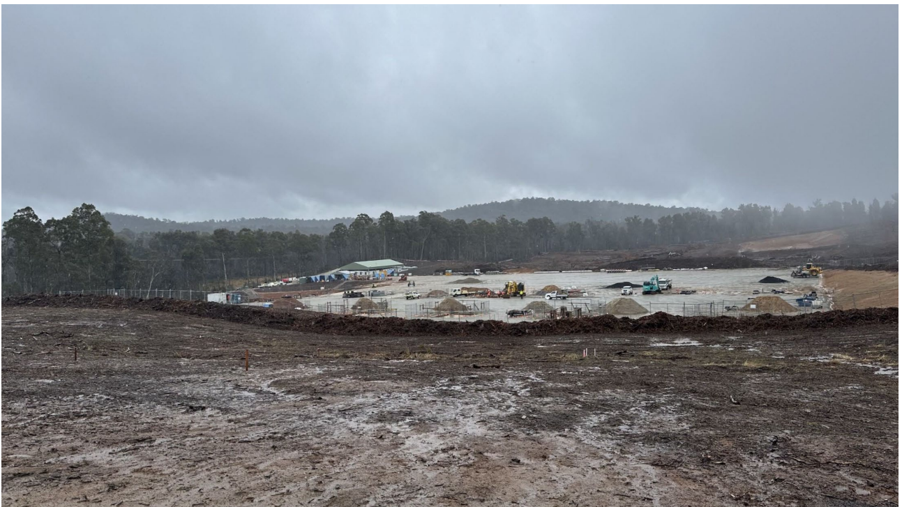
Plate 13: Sediment basin located within Maragle Substation Project Area (25/09/2024).
