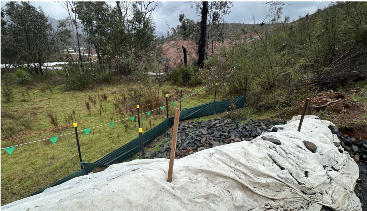
Plate 5: Erosion and sediment control devices e.g. coir logs installed alongside roadside (25/09/2024).
