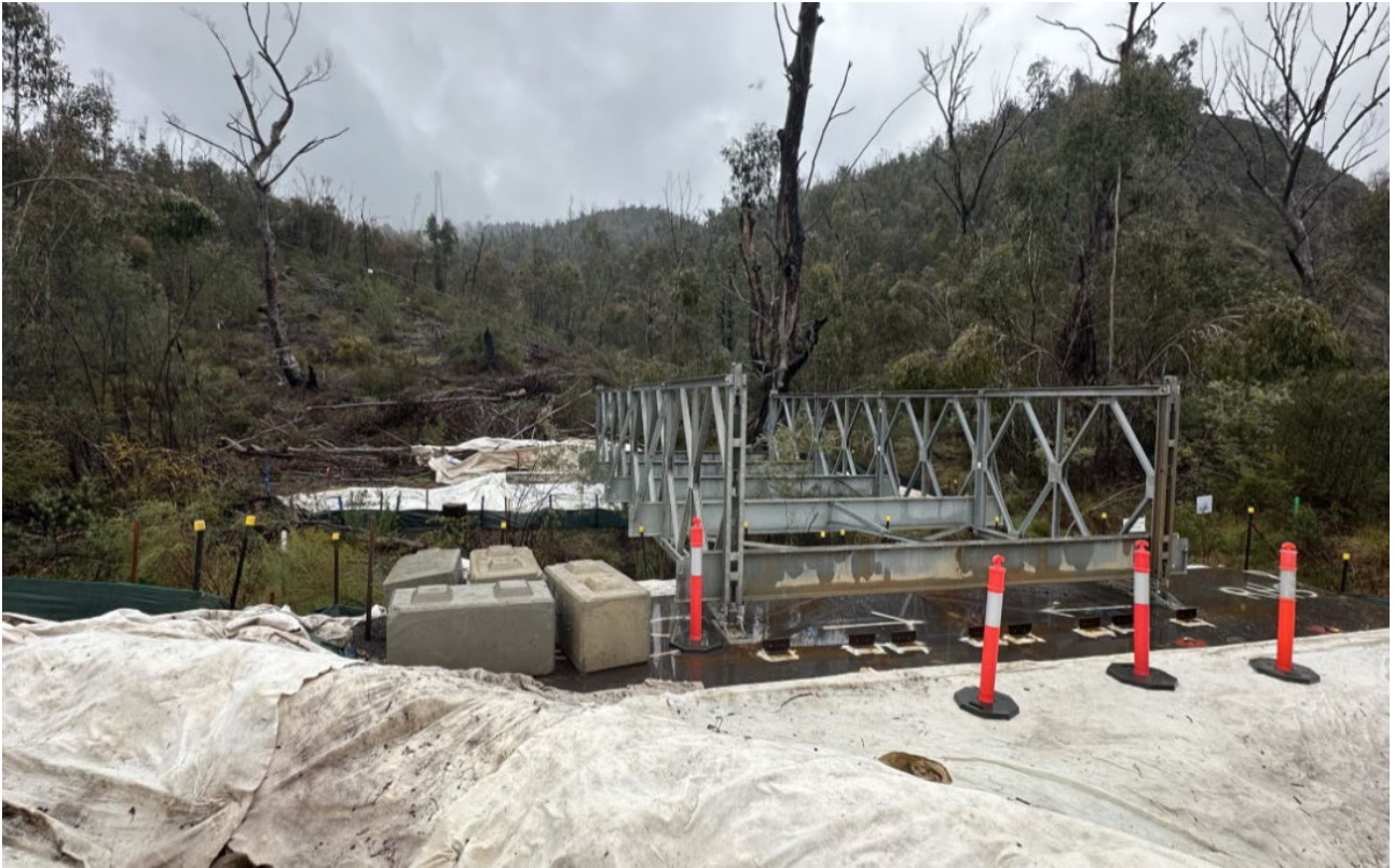
Plate 23: An overview of the temporary bridge located at Sheep Station Creek (25/09/2024).
