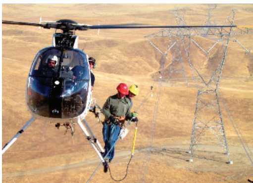
FireFly FF can be installed by helicopter
