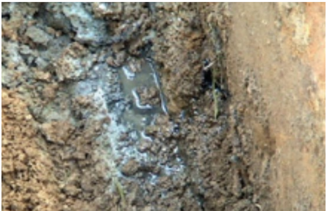
Excavation reveals oil contamination in an excavation next to a Transformer Bund
