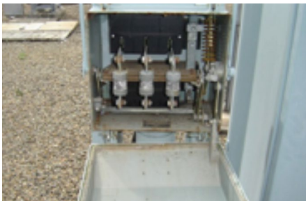
ACM rope seals of fuse box
