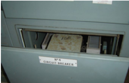
ACM asbestos arc shields
