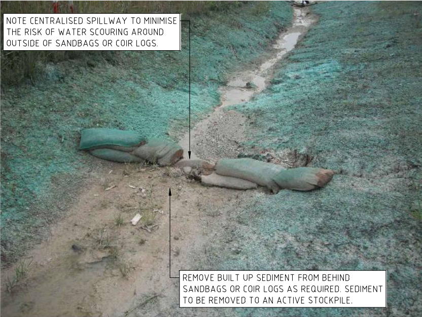
PHOTO 2: EXAMPLE OF CHECK DAM WITH CENTRALISED SPILLWAY.
